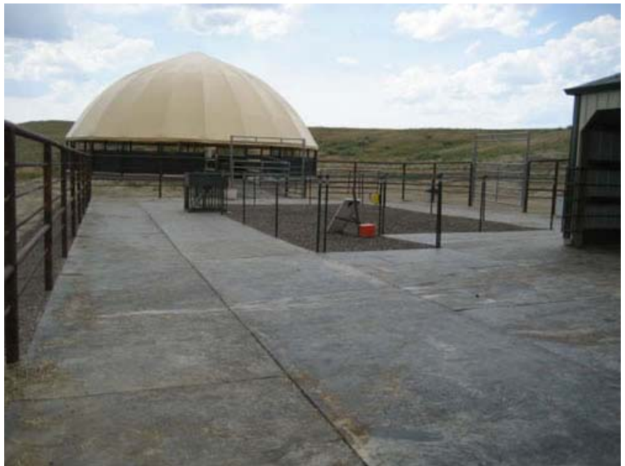
Rubber floor and the covered 6 horse walker are the center of the Wyoming Lameness Center
